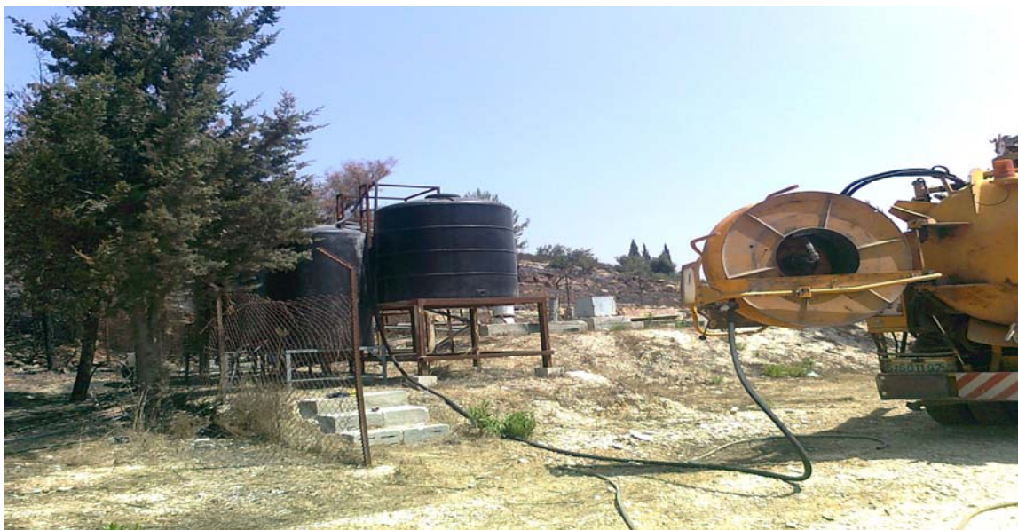
Figure 3-5: Treated wastewater transporting and storing.
