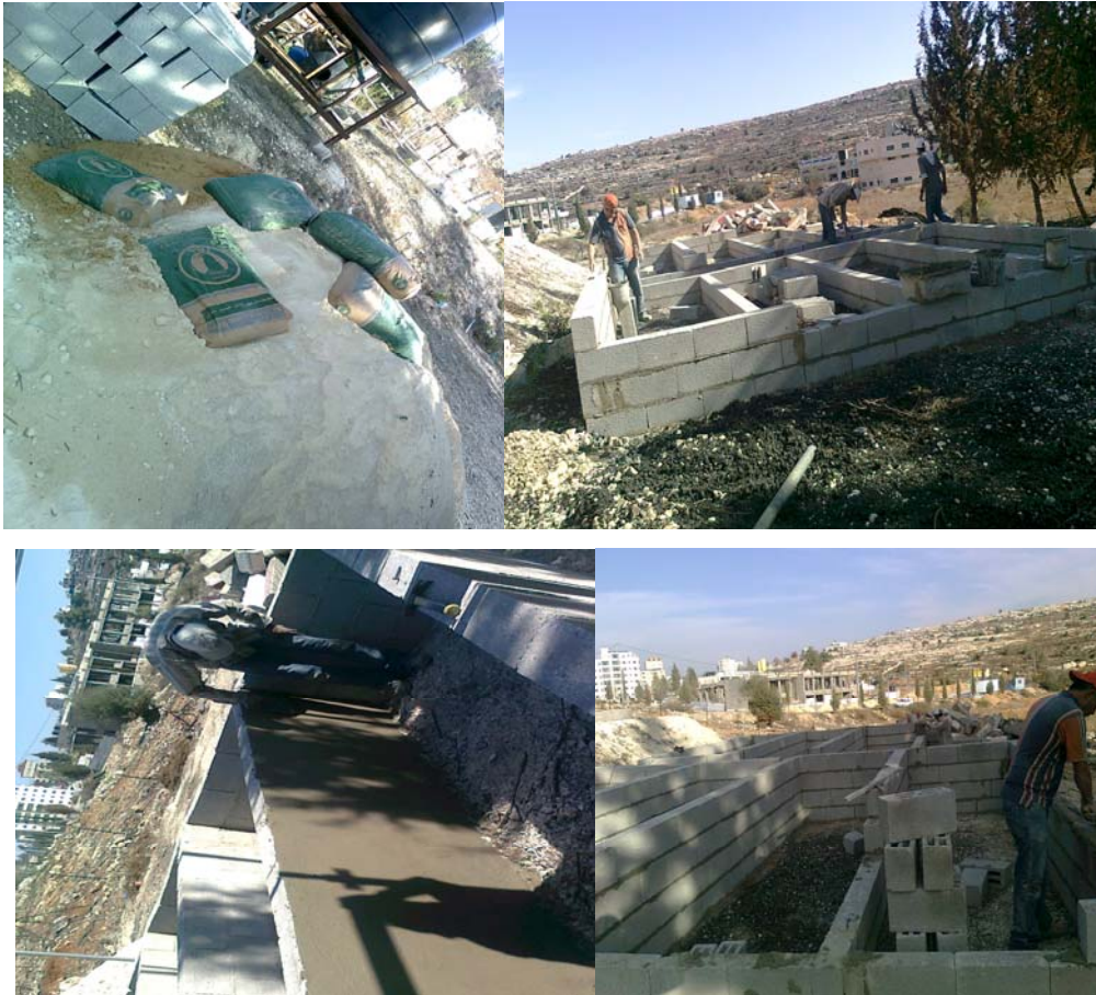
Figure 3-3: Agricultural docks building works.
